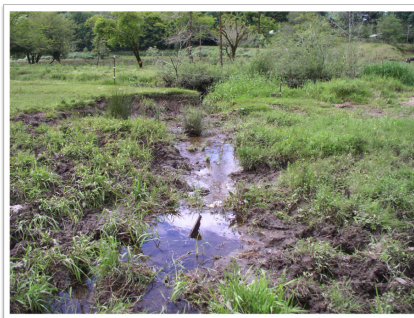
Ditch in need of improvement
